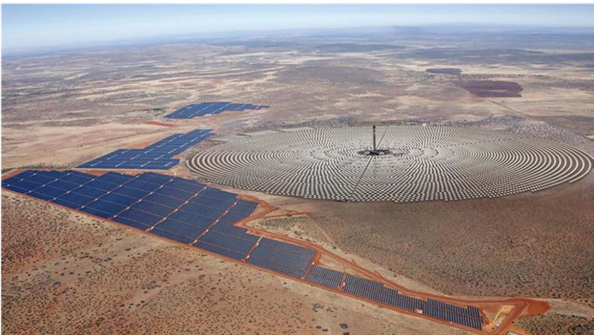
For example : an existing 160 MW of PV (Photo Voltaic) Solar Power facility & proposed 100 MW CSP (Concentrating Solar-thermal Power) project in the Northern Cape Province, South Africa by Solar Reserve.
